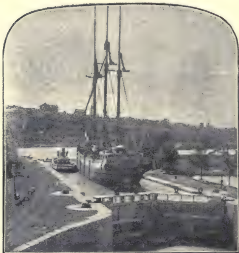
FIG. 43—The Welland Canal, showing a lock with vessel passing from Lake Ontario to Lake Erie
